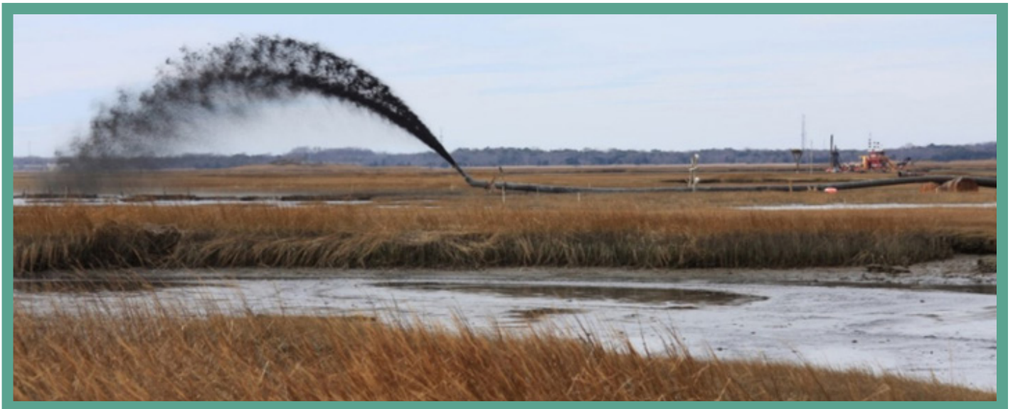
Figure 20. TLP by Conventional Cutterhead with a Crib-Mounted High-Pressure Nozzle at Avalon, New Jersey (Source: New Jersey Department of Transportation [NJDOT], Office of Maritime Resources [OMR])
