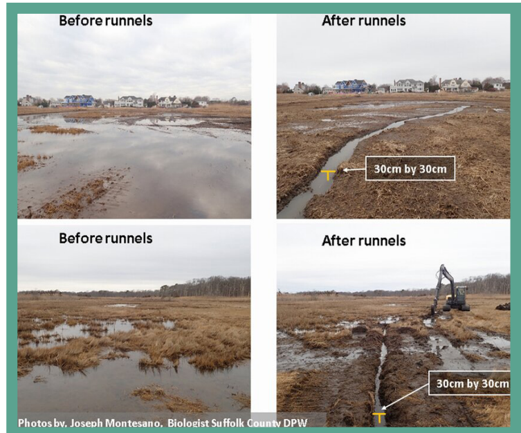
Tidal creek restoration using runnels (Source: Suffolk County DPW)
