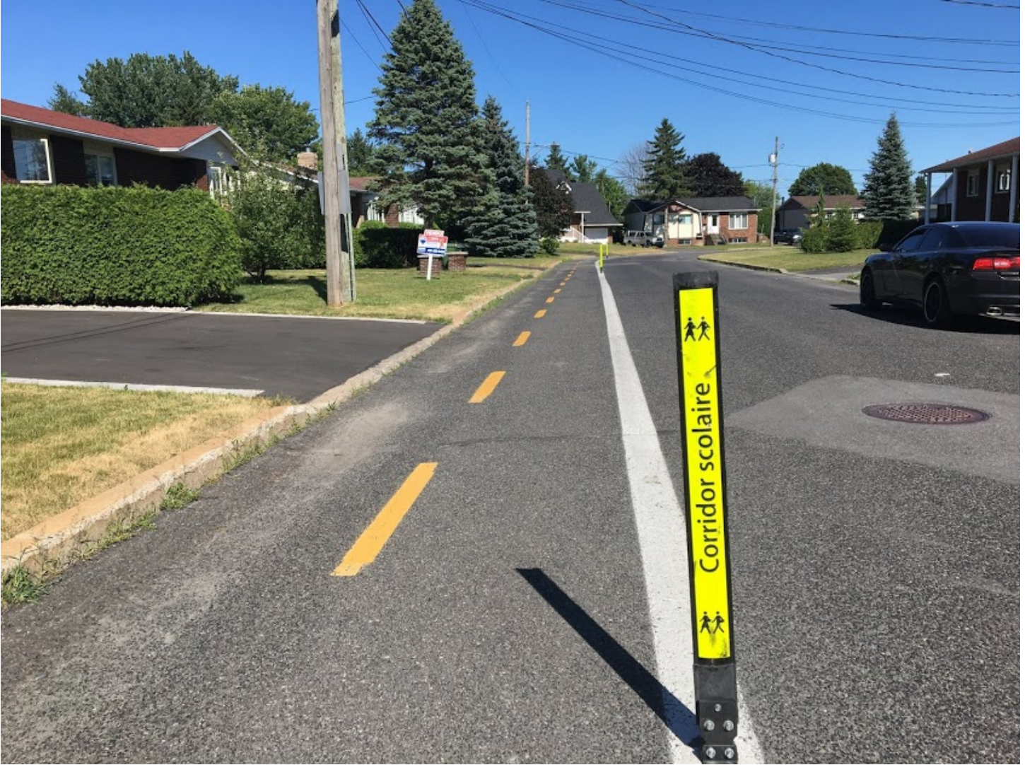
Fig. 10 Example On-street Bike/Walk facilities
