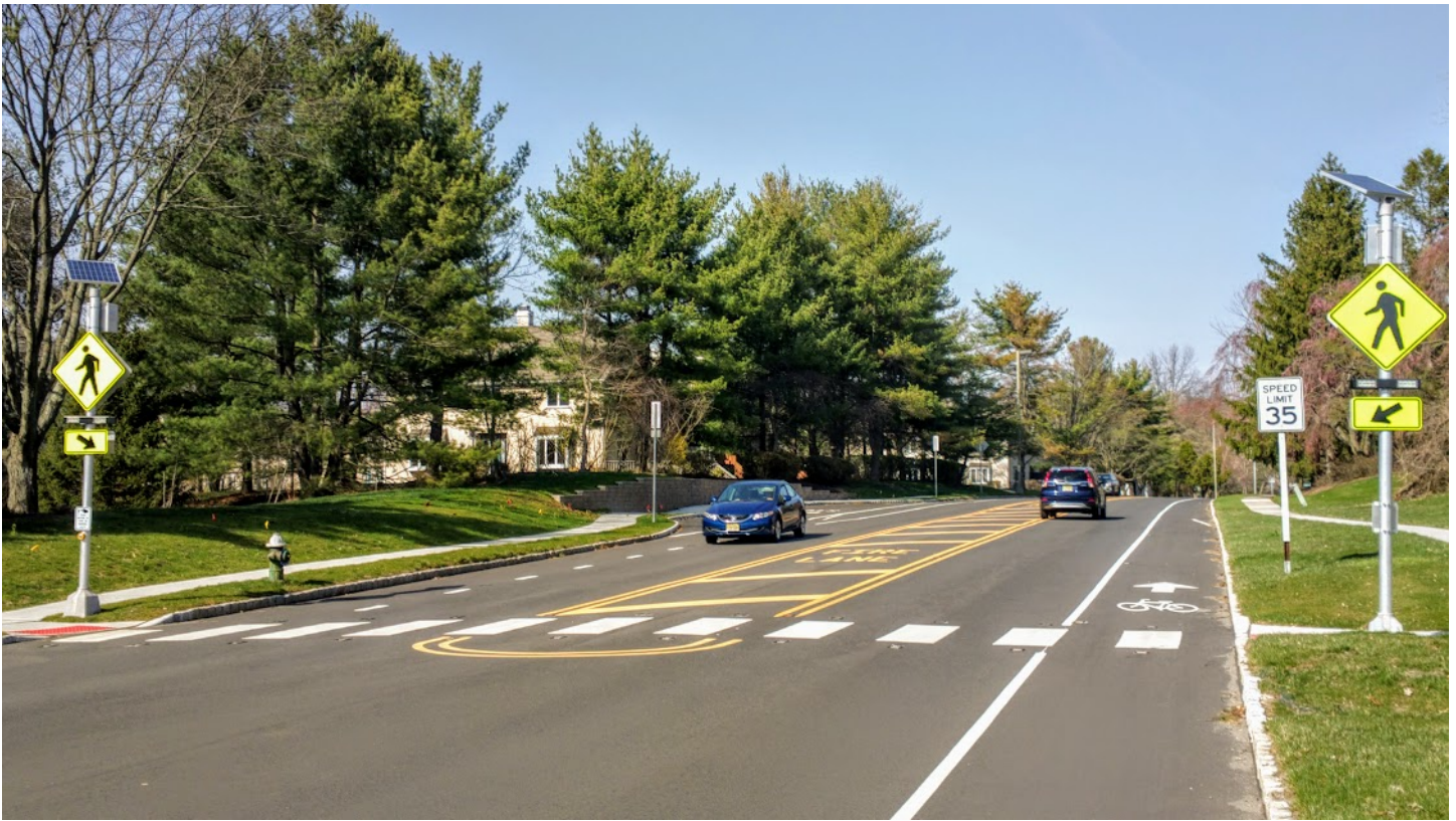
Fig 12 Example Pedestrian Crossing - Rectangular Rapid-Flashing Beacon
