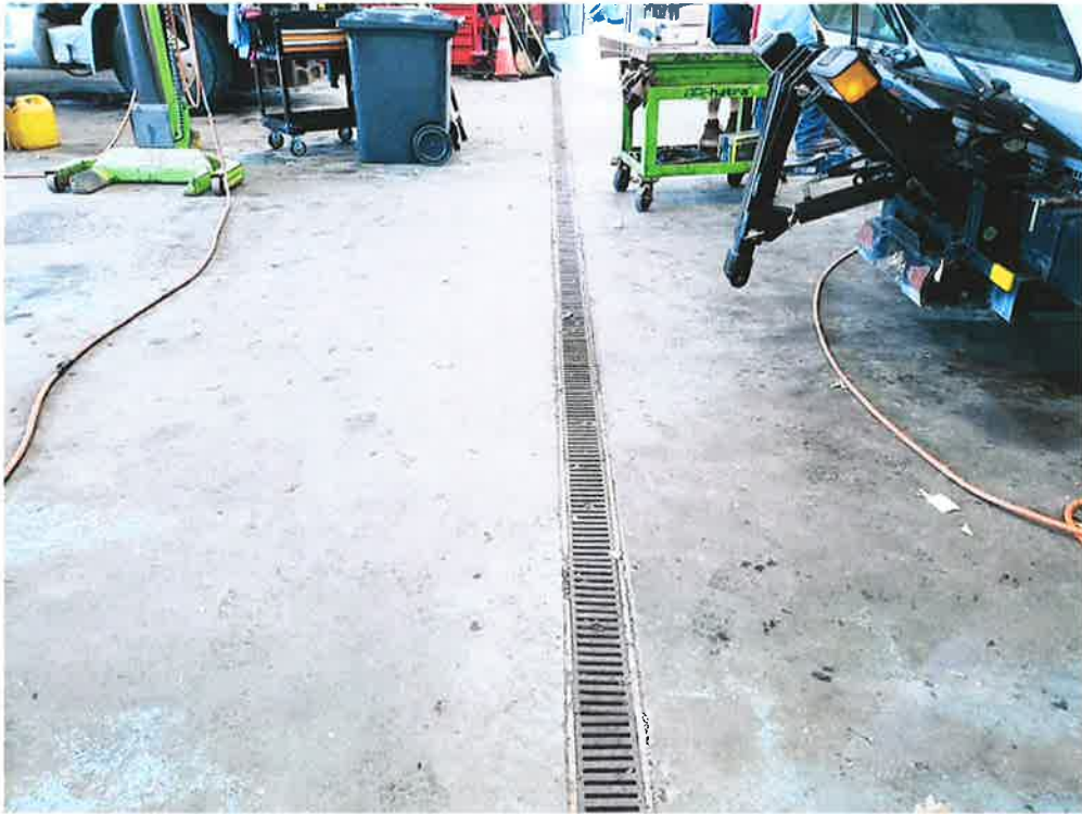
Floor Drain within Garage
