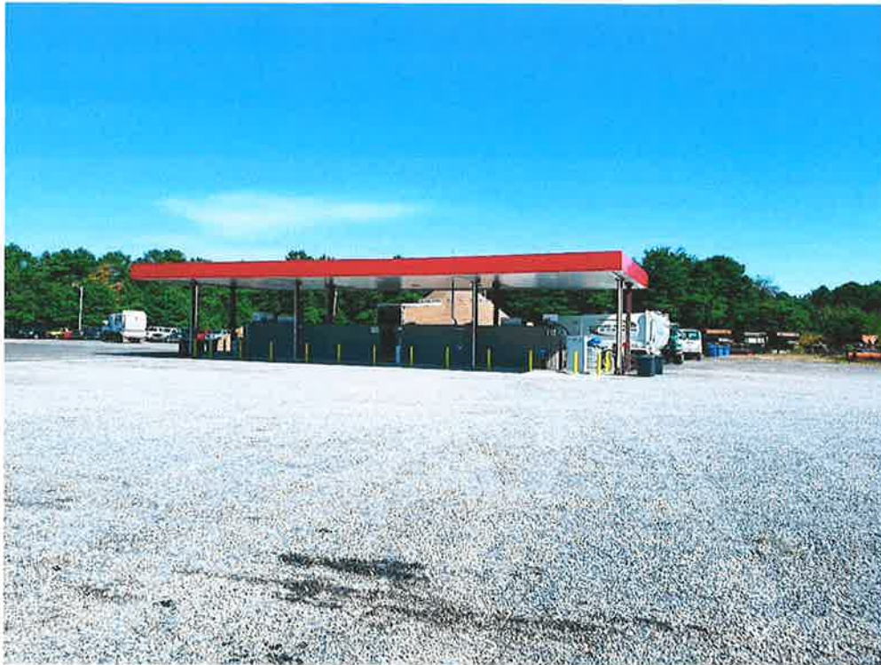
AST 1: 12,000-gal Gasoline & AST 2: 12,000-gal Diesel Fuel
