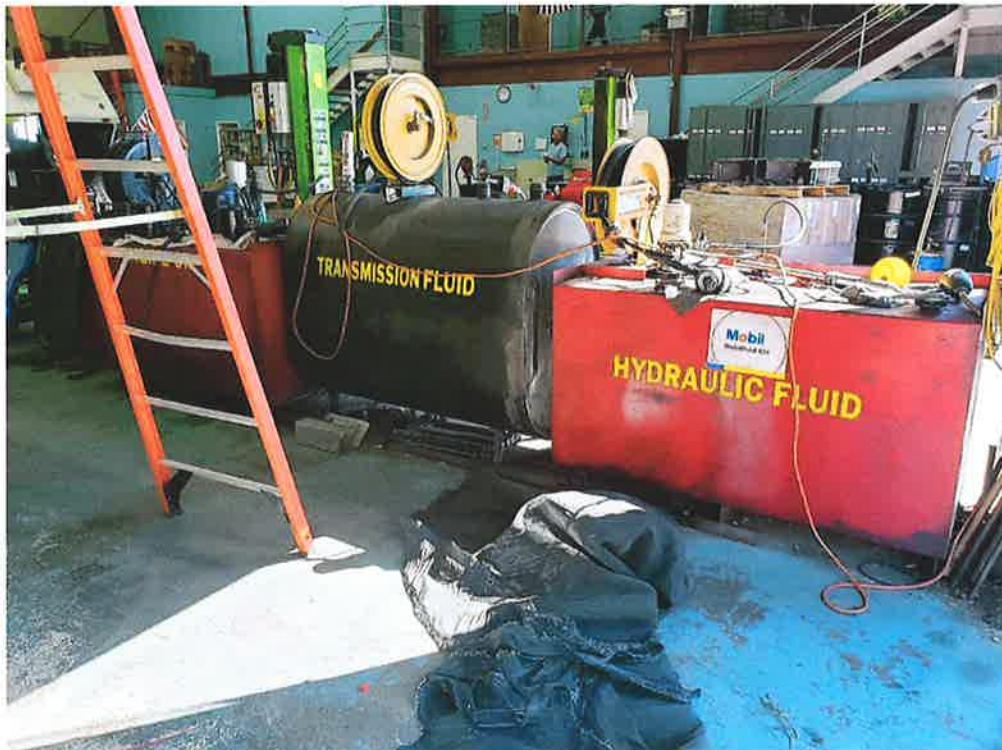
AST 5: 300-gal Hydraulic Fluid; AST 6: 300-gal Transmission Fluid; AST 7: 300-gal Motor Oil
